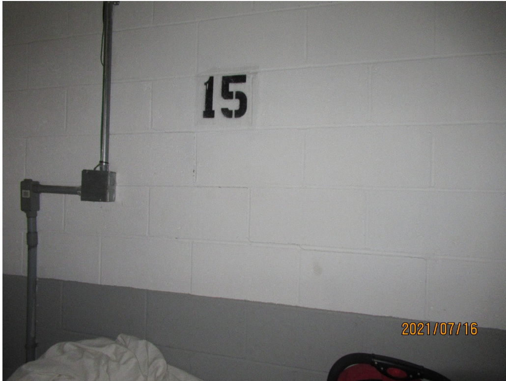
Figure 5. Minor Step Cracking at Masonry Block Exterior Wall at Northwest Building Corner
