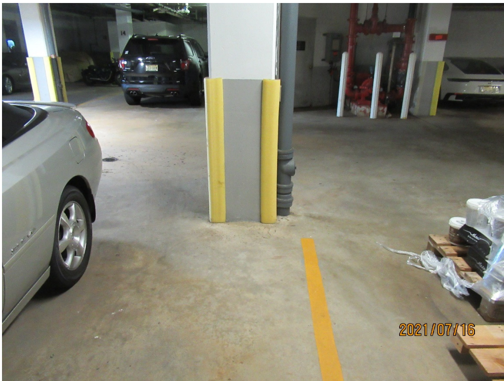
Figure 4. Typical Concrete Column at Ground Level Grade Supported Slab
